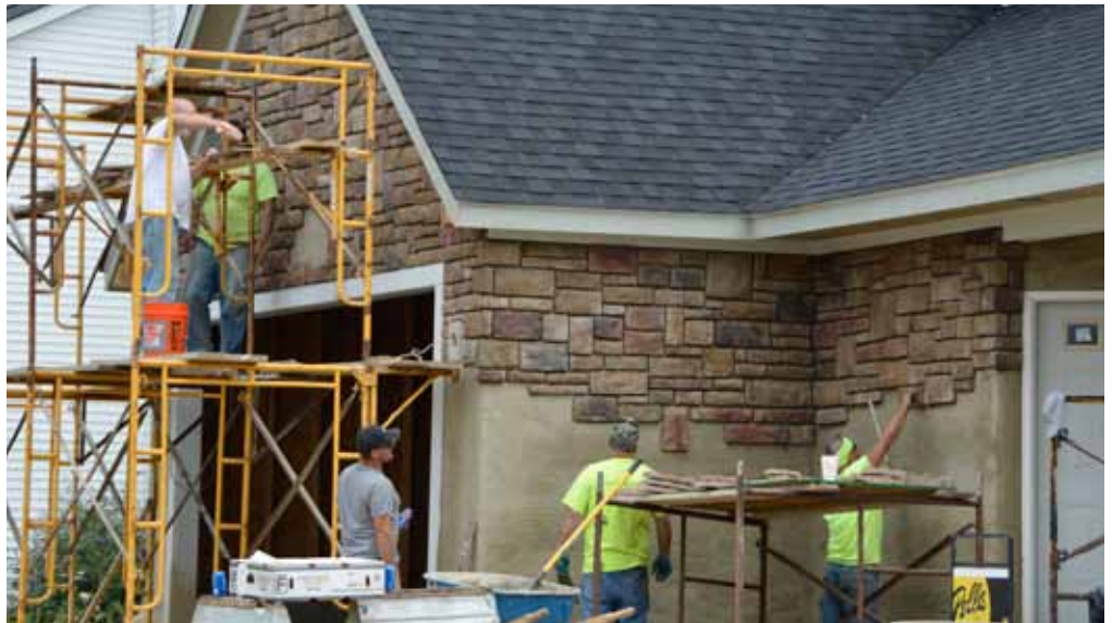
PHOTOS: COURTESY OF LOCAL 55
